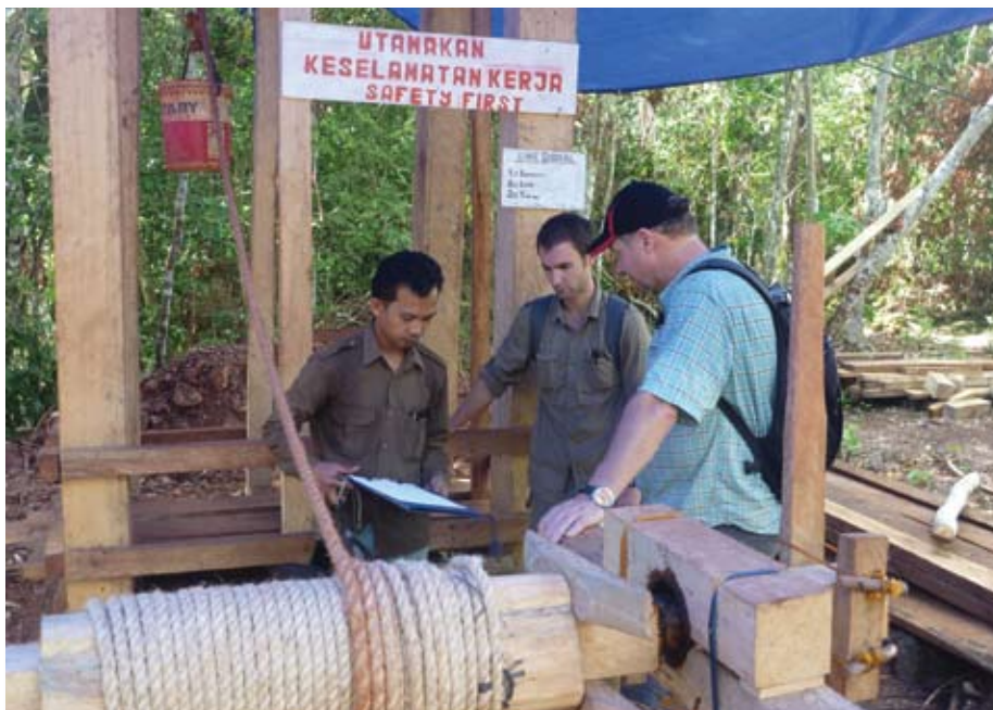
Shaft construction at Batu Hitam, Lakuwahi Prospect
